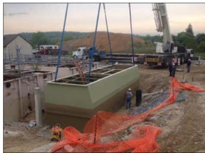
**Equalization Tank Repair** – All that remains of this emergency repair that began in January is the installation of the walkway. While these expenses were unexpected, the repair work included improvements to the plant property and should extend the life of the Equalization Tank. We are happy to have this project mostly behind us and the plant operating more efficiently.
