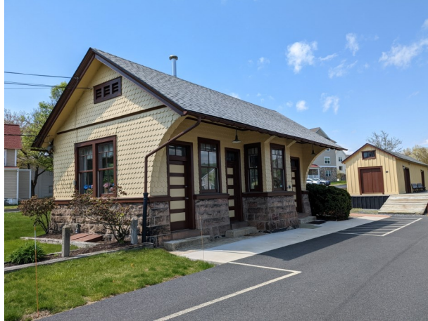
The Elverson Railroad Station today.
