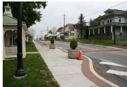
A view of the recent improvements created with the Main Street Streetscape project, including crosswalks, a bump-out, and on-street parking.
